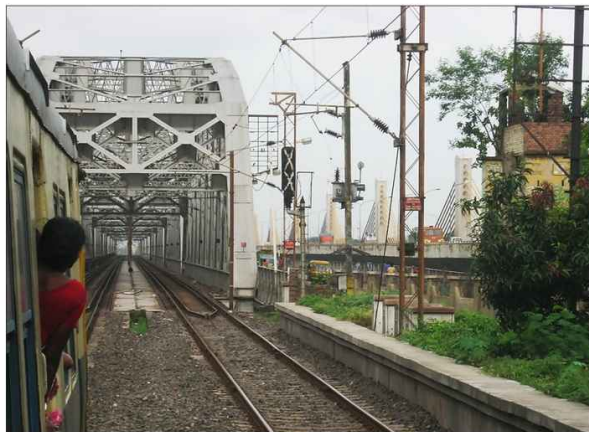
An EMU Train Entering the Mighty Rail-cum-Road Bally Bridge
