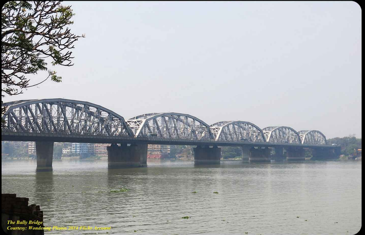
The Road-cum-Rail Bally Bridge aka Vivekananda Setu Courtesy: Rudranil Roy Chowdhury
