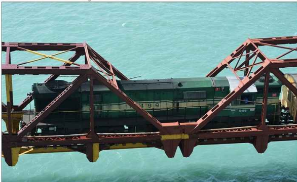
A train on the double-leaf bascule section...
