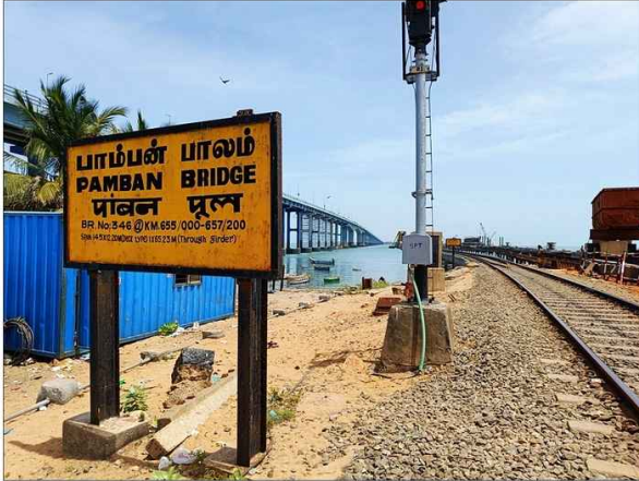
The Pamban Bridge entrance...
