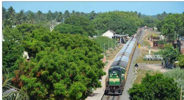
An aerial view of Pamban station...
