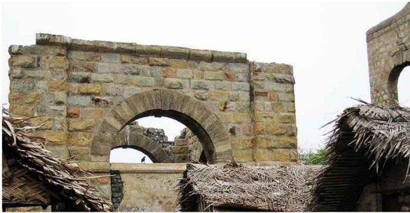
Masonry structures of old Dhanushkodi station
