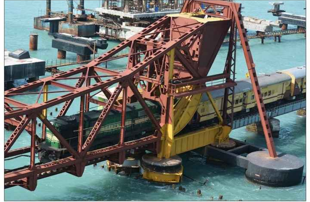
The Bascule section of iconic Pamban bridge..
