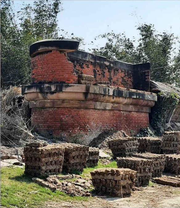
Abutment (East Bank) from Front Side
