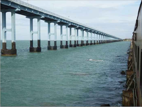
Annai Indira Gandhi Road bridge view from Pamban bridge.
