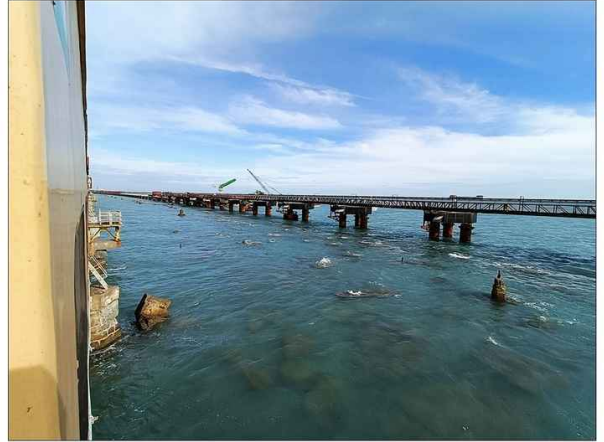
The new Pamban railway bridge coming up...
