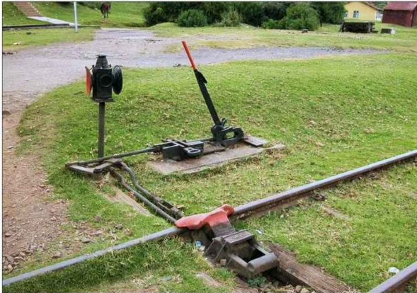
The unique derailing point in Ooty station...
