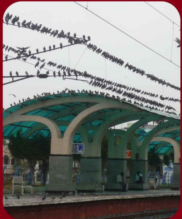
Necklace Road station is home to a flock of pigeons & they are accustomed to the MMTS EMUs.
