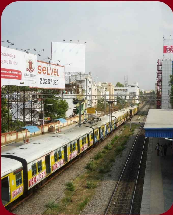
The afternoon service from Falaknuma to Nampally is seen here departing from Khairatabad station. This station existed before the MMTS era and had a loop line between the two tracks which was later removed. (15 May 2013)
