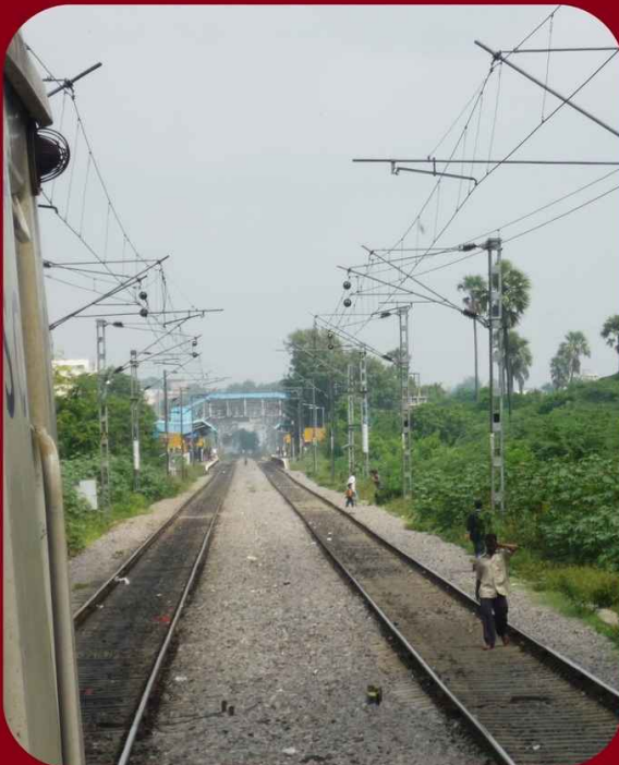
If you stop at Jama-i-Osmania station and look towards Secunderabad, you will be able to see the very next station - Arts College at a distance. The two stations are roughly a kilometer apart. If you look closely, you can also spot a part of the velodrome next to the Arts College station.
