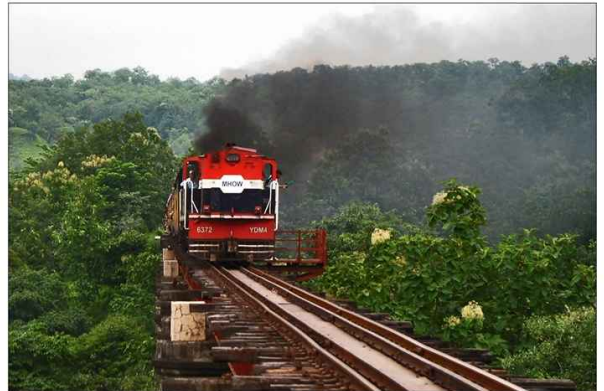
470 Dn over the viaduct
