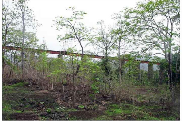
Long view of the Dhulghat viaduct
