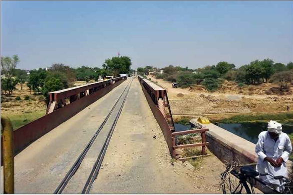
Road-cum-rail bridge over Kauri river
