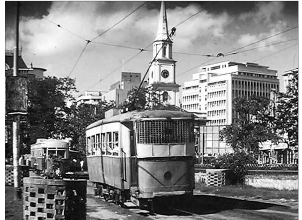
Converted unidirectional single cars joined to form double coach tram
