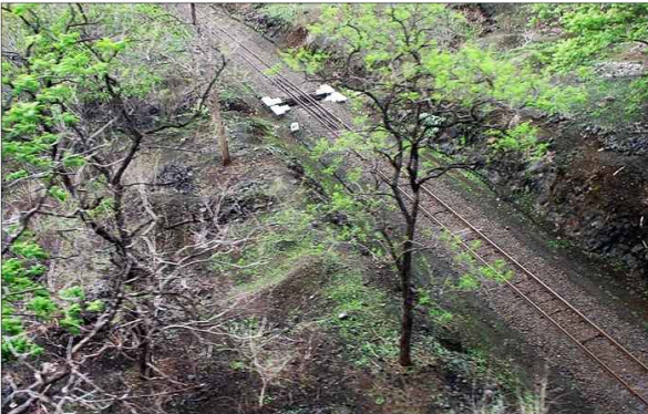
The view of the spiral from the viaduct
