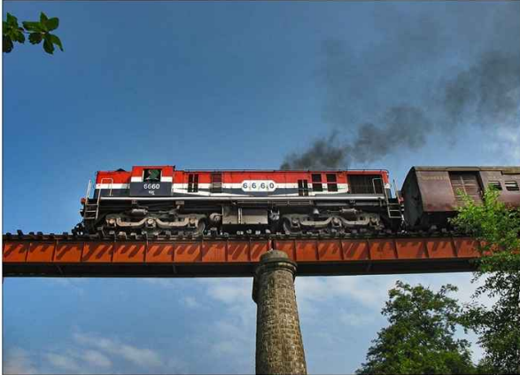
457 Passenger passing over the viaduct
