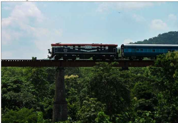
458B Passenger over the viaduct
