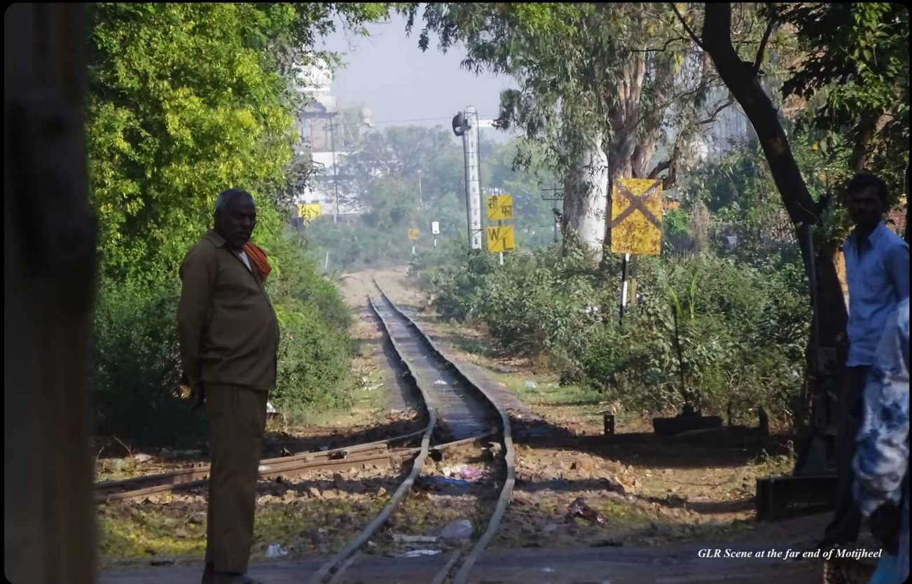
Train halted due to a minor derailment at Fort Road
