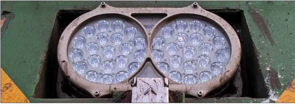
WAG9H # 31628 fitted with LED Twin Beam Setup replacing regular PAR56/MFL lamps
