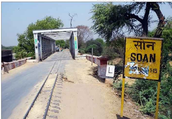
Road-cum-rail bridge over the river Soan
