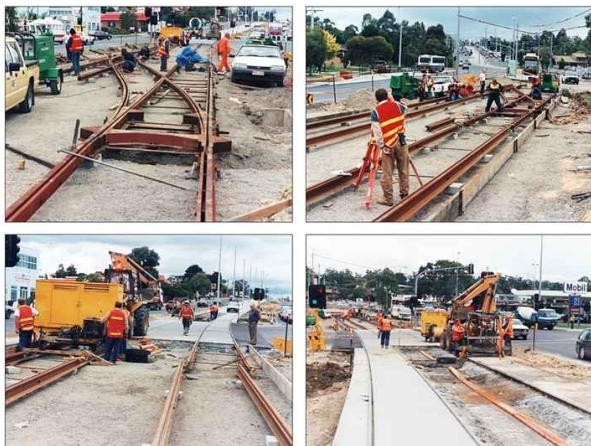
▲ Tram tracks renewal works at Melbourne
