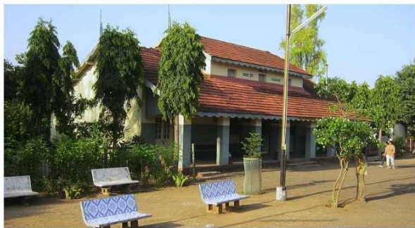
Sasan Gir Station
