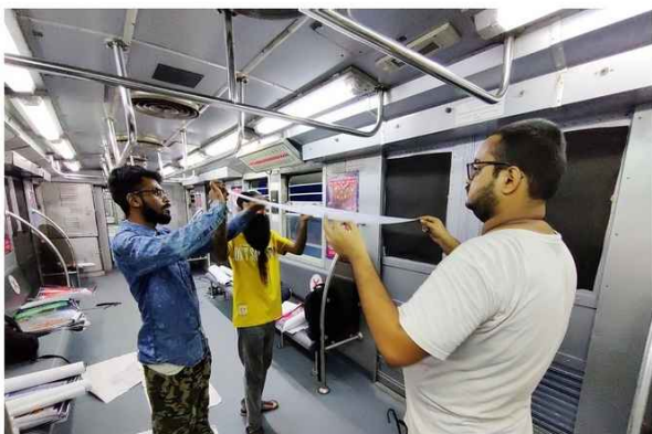
Work in full swing
