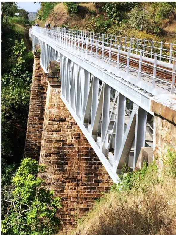
Ravine Viaduct No. 1
