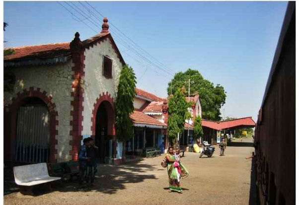
The Railway settlement @ Amreli
