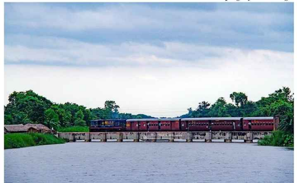
Gopalganj Rail Bridge
