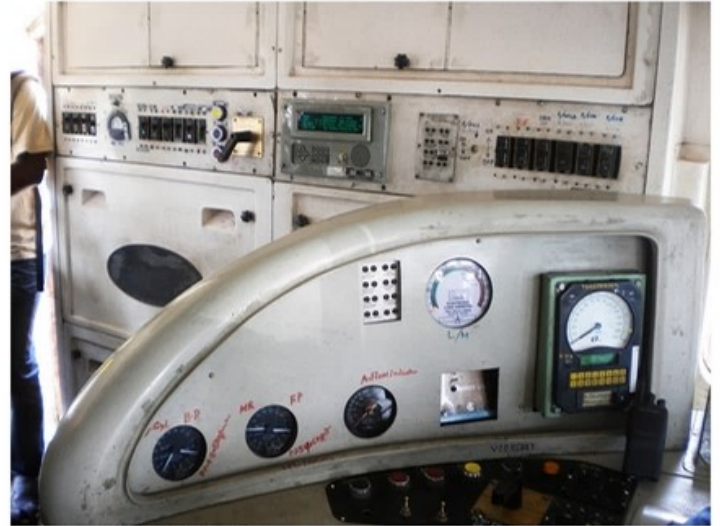
Driving Panel of WDM2/3A Locomotive
