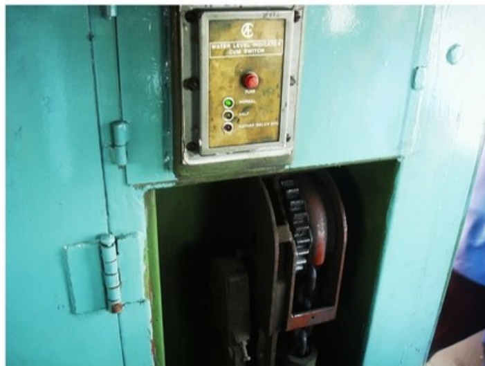
Water Level Indicator inside a BG Diesel Locomotive
