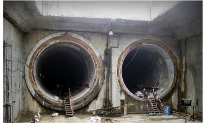
Howrah end of underwater twin tunnels
