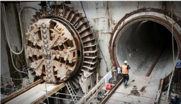
Rotating cutter-head of a TBM
