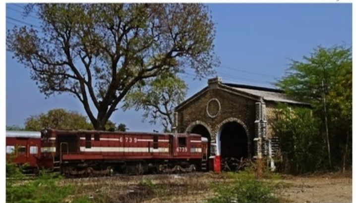
Diesel Locomotive Shed - Mavli Jn.
