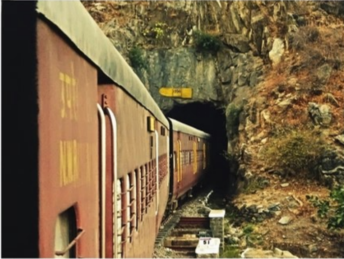
Tunnel dates back to 1934
